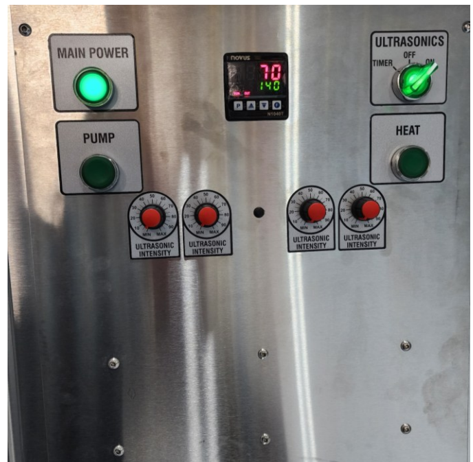
Figure 11: Generator Manual Control On
