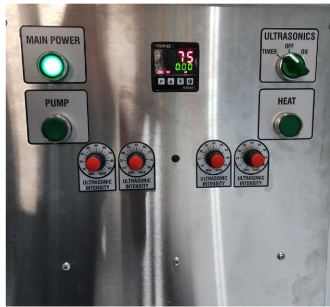
Figure 16: Generator Timer Cycle Done
