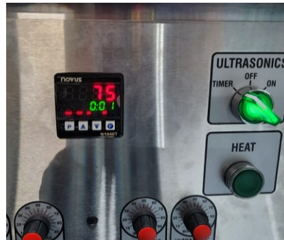
Figure 13: Generator Timer Running
